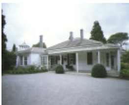
the heights 140 aphrasia street geelong exterior view
