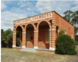
FORMER HUNTLY SHIRE COUNCIL CHAMBERS SOHE 2008
