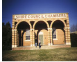
1 former huntly shire council chambers front view jun1997
