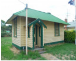
FORMER NEWSTEAD SHIRE CHAMBERS SOHE 2008
