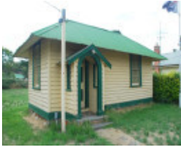
FORMER NEWSTEAD SHIRE CHAMBERS SOHE 2008
