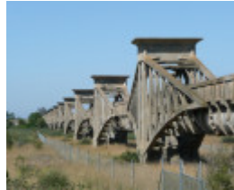
OVOID SEWER AQUEDUCT OVER BARWON RIVER SOHE 2008
