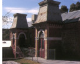
1 fuse factory bendigo side view
