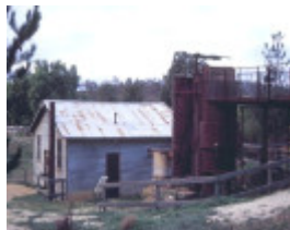
h01322 1 forest creek tourist gold mine castlemaine and chewton road castlemaine engine shed side elevation she project 2003
