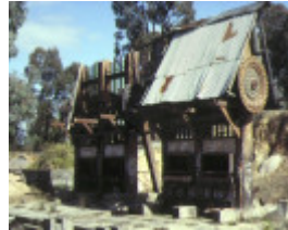
1 victoria hill mines bendigo machinery ruins
