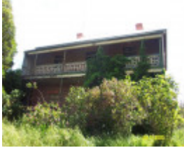
52787 Nangeela Homestead Casterton facade 245
