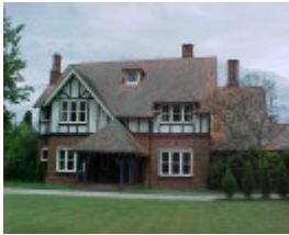
H01399 residence formerly colinton mont albert road canterbury front view nov2001
