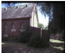
st pauls church of england geelong kindergarten hall
