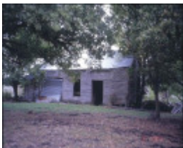
h01387 timboon house old geelong road camperdown original stables she project 2003
