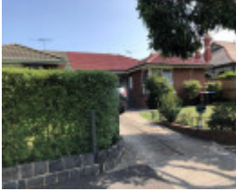
84 Claremont Avenue, Malvern
