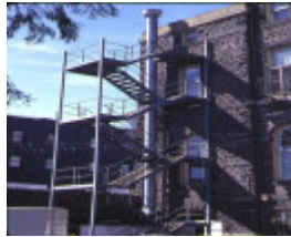
former es&a bank malop street geelong fire escape
