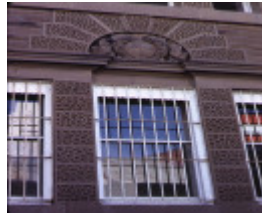
former es&a bank malop street geelong detail external window
