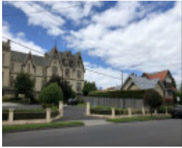
Maud Street elevation with bungalow at right
