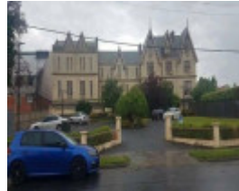
Maud Street Entrance
