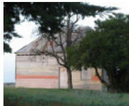
Residence Stawell Street Tarraville
