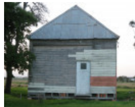
Residence Stawell Street Tarraville
