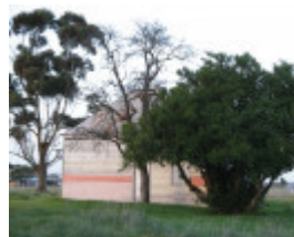
Residence Stawell Street Tarraville
