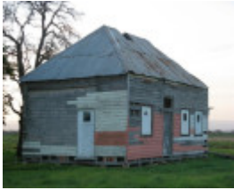
Residence Stawell Street Tarraville small
