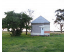
Residence Stawell Street Tarraville
