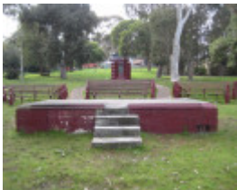
Before Photograph - Reference F3921 2014
