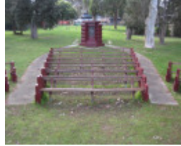
Before Photograph - Reference F3921 2014
