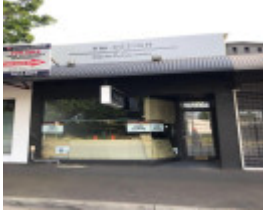
119 Station Street, Malvern
