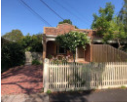
36 Victoria Road North, Malvern
