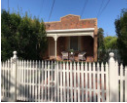
38A Victoria Road North, Malvern
