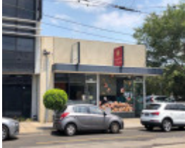
148-150 Wattletree Road, Malvern
