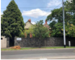
198 Wattletree Road, Malvern
