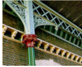
geelong railway station & goods shed railway terrace geelong roof detail publication
