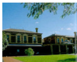
geelong railway station & goods shed railway terrace geelong verandah view publication
