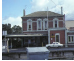
geelong railway station & goods shed geelong side view
