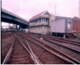
Geelong Railway Station Signal Box
