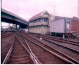
Geelong Railway Station Signal Box
