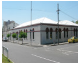
FORMER MELBOURNE OMNIBUS COMPANYS STABLES SOHE 2008
