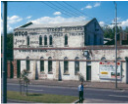
h01810 1 melbourne omnibus building 1997
