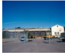
h01810 2 melbourne omnibus building 1997
