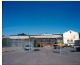
h01810 2 Melbourne omnibus building 1997
