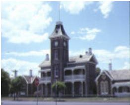
austin hall & terrace complex yarra & mundy streets south geelong front view of austin hall jan1997
