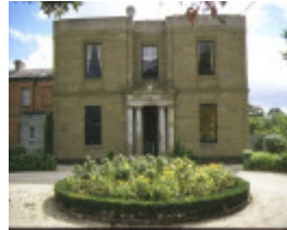
1 lunan house geelong west front elevation lunan house apr1997
