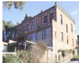
h01774 186 192 clarke street northcote rear elevation sep1998
