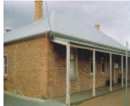
former harp inn packington street geelong west verandah view publication
