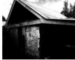
Detached store or early house from the south-east, showing shingle roof under added gabled roof
