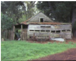
silverwells gembrook former post office & store
