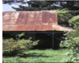
silverwells gembrook front entrance to third house oct1980
