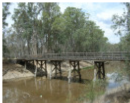
CONDIDORIOS BRIDGE SOHE 2008
