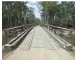
CONDIDORIOS BRIDGE SOHE 2008
