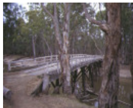
1 condidorios bridge koondrook
