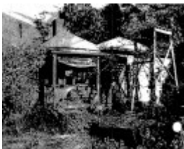
12.11 - Tregowan Cottage 06 - Shire of Whittlesea Heritage Study 1991
