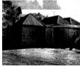
12.11 - Tregowan Cottage 02 - Shire of Whittlesea Heritage Study 1991
