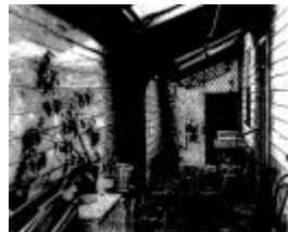
12.11 - Tregowan Cottage 04 - Shire of Whittlesea Heritage Study 1991
