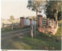
2 - Maroondah Aqueduct Kangaroo Ground Eltham - Shire of Eltham Heritage Study 1992 - Colour 7
