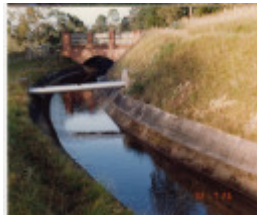
2 - Maroondah Aqueduct Kangaroo Ground Eltham - Shire of Eltham Heritage Study 1992 - Colour 5
