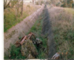
2 - Maroondah Aqueduct Kangaroo Ground Eltham - Shire of Eltham Heritage Study 1992 - Colour 11
