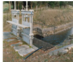
2 - Maroondah Aqueduct Kangaroo Ground Eltham - Shire of Eltham Heritage Study 1992 - Colour 3
