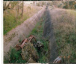
2 - Maroondah Aqueduct Kangaroo Ground Eltham - Shire of Eltham Heritage Study 1992 - Colour 11
