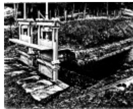
2 - Maroondah Aqueduct Kangaroo Ground Eltham N04 - Shire of Eltham Heritage Study 1992 - Western End of the above mentioned syphon discharging into a section of open aqueduct
