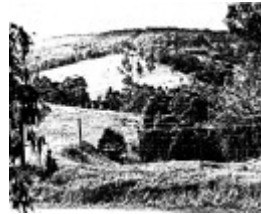
2 - Maroondah Aqueduct Kangaroo Ground Eltham N02 - Shire of Eltham Heritage Study 1992 - Inverted syphon across Watsons Creek, one of fourteen totalling 14.88 km of the 65.97 km total length of the Maroondah Aqueduct
