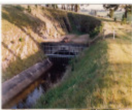
2 - Maroondah Aqueduct Kangaroo Ground Eltham - Shire of Eltham Heritage Study 1992 - Colour 4
