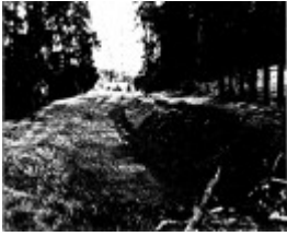
2 - Maroondah Aqueduct Kangaroo Ground Eltham N15 - of Eltham Heritage Study 1992 - Section of Aqueduct at Research that has been removed/filled in and replaced by a pipeline. A tunnel began/begins here. The surviving radiata pine tree plantings
