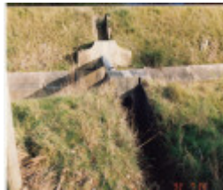
2 - Maroondah Aqueduct Kangaroo Ground Eltham - Shire of Eltham Heritage Study 1992 - Colour 6
