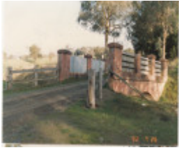
2 - Maroondah Aqueduct Kangaroo Ground Eltham - Shire of Eltham Heritage Study 1992 - Colour 7
