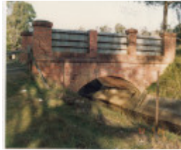
2 - Maroondah Aqueduct Kangaroo Ground Eltham - Shire of Eltham Heritage Study 1992 - Colour 8
