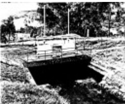
2 - Maroondah Aqueduct Kangaroo Ground Eltham N03 - Shire of Eltham Heritage Study 1992 - Inverted syphon across Watsons Creek, one of fourteen totalling 14.88 km of the 65.97 km total length of the Maroondah Aqueduct
