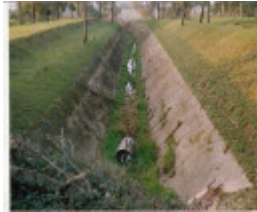
2 - Maroondah Aqueduct Kangaroo Ground Eltham - Shire of Eltham Heritage Study 1992 - Colour 10
