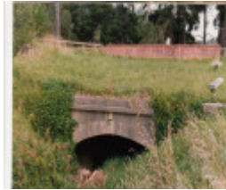
2 - Maroondah Aqueduct Kangaroo Ground Eltham - Shire of Eltham Heritage Study 1992 - Colour 9
