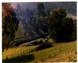
2 - Maroondah Aqueduct Kangaroo Ground Eltham - Shire of Eltham Heritage Study 1992 - Grassy hill
