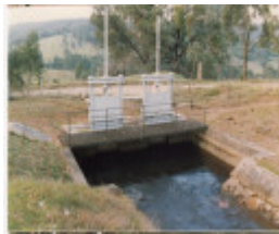
2 - Maroondah Aqueduct Kangaroo Ground Eltham - Shire of Eltham Heritage Study 1992 - Colour 2
