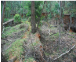
YACKANDANDAH CREEK GOLD HYDRAULIC SLUICING WORKS SOHE 2008
