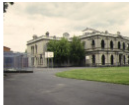
1 malvern house willoby ave glen iris front view property 1994
