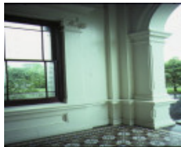
malvern house willoby ave glen iris interior tiled floor nov1985
