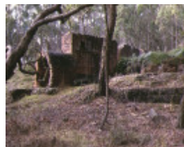
1 jubilee company quartz gold mine near newtown battery engine compressor apr1998
