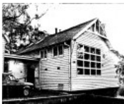
10 - Scouts Building Former State School 3939_02 - Shire of Eltham Heritage Study 1992
