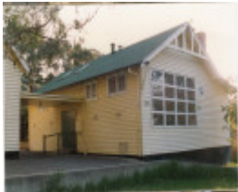
Scouts Building Former State School 3939 Colour 1 - Shire of Eltham Heritage Study 1992
