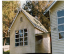
Scouts Building Former State School 3939 Colour 3 - Shire of Eltham Heritage Study 1992
