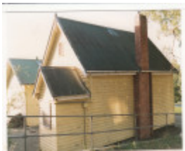
Scouts Building Former State School 3939 Colour 4 - Shire of Eltham Heritage Study 1992
