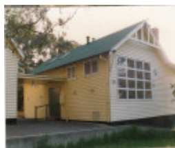
Scouts Building Former State School 3939 Colour 1 - Shire of Eltham Heritage Study 1992
