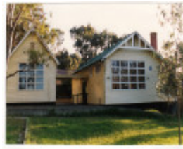
Scouts Building Former State School 3939 Colour 2 - Shire of Eltham Heritage Study 1992
