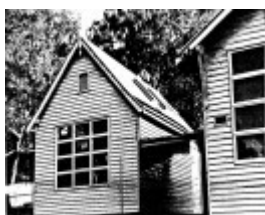
10 - Scouts Building Former State School 3939_03 - Shire of Eltham Heritage Study 1992
