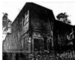
18 - Frank Werther Residence off Barreenong Rd - Shire of Eltham Heritage Study 1992
