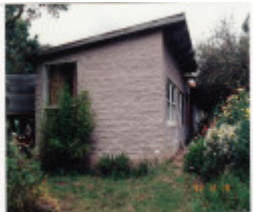
Alma Shanahan Adobe Residence 135 Barreenong Rd Colour 4 - Shire of Eltham Heritage Study 1992
