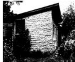
21 - Alma Shanahan Adobe Residence 135 Barreenong Rd_02 - Shire of Eltham Heritage Study 1992
