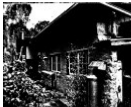
21 - Alma Shanahan Adobe Residence 135 Barreenong Rd_04 - Shire of Eltham Heritage Study 1992
