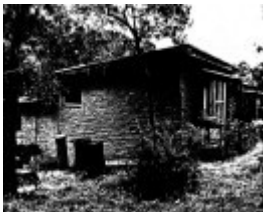
21 - Alma Shanahan Adobe Residence 135 Barreenong Rd_03 - Shire of Eltham Heritage Study 1992
