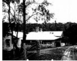
27 - Walter Withers House - Southernwood 250 Bolton St_02 - Shire of Eltham Heritage Study 1992
