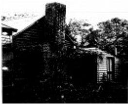
27 - Walter Withers House - Southernwood 250 Bolton St_04 - Shire of Eltham Heritage Study 1992
