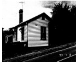
27 - Walter Withers House - Southernwood 250 Bolton St_06 - Shire of Eltham Heritage Study 1992
