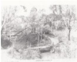
Timber Trestle Road Bridge over Diamond Creek Wooden Bridge - Shire of Eltham Heritage Study 1992
