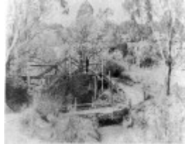
29 - Timber Trestle Road Bridge over Diamond Creek - Similar Bridge over Diamond Creek photographed during the early/mid 20th Century - Shire of Eltham Heritage Study 1992
