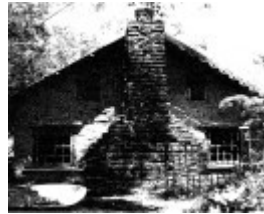
30 - Peter Garner MudBrickStudio andShed 62 Brougham St_02 - Shire of Eltham Heritage Study 1992
