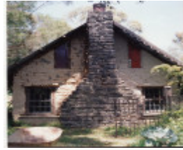
Peter Garner Mud Brick Studio and Shed 62 Brougham St Colour 8 - Shire of Eltham Heritage Study 1992
