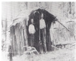
Miners Timber Slab Cottage 2 Castle Rd Black & White - Shire of Eltham Heritage Study 1992
