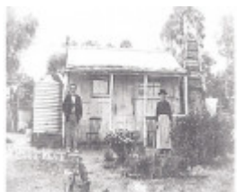
Miners Timber Slab Cottage 2 Castle Rd Black & White 3 - Shire of Eltham Heritage Study 1992
