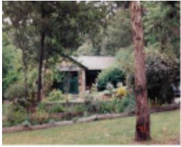
Florries Cottage 28 30 Diamond St Colour 1 - Shire of Eltham Heritage Study 1992
