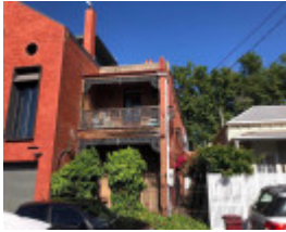
7A Stuart Street, Armadale
