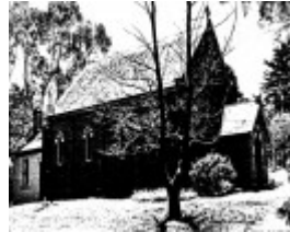
63 - Presbyterian Church Eltham Yarra Glen Rd_02 - Shire of Eltham Heritage Study 1992
