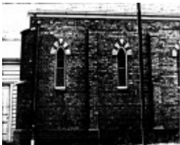
63 - Presbyterian Church Eltham Yarra Glen Rd_04 - Shire of Eltham Heritage Study 1992
