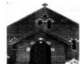
63 - Presbyterian Church Eltham Yarra Glen Rd_08 - Shire of Eltham Heritage Study 1992
