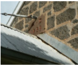
Teesdale Presbyterian Church, Pyke Street Teesdale
