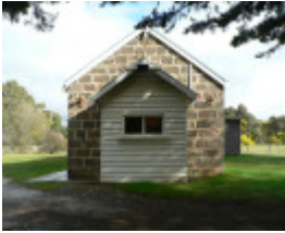
Teesdale Presbyterian Church, Pyke Street Teesdale
