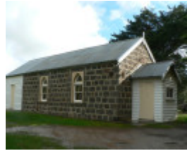
Teesdale Presbyterian Church, Pyke Street Teesdale
