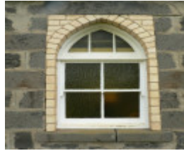
Teesdale Presbyterian Church, Pyke Street Teesdale
