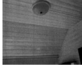
Early chamfered ceilings under gabled wings - Shire of Nillumbik Study, 2000
