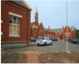
PRIMARY SCHOOL NO. 1566 SOHE 2008
