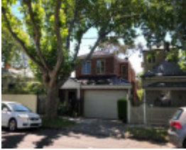
37 Union Street, Armadale
