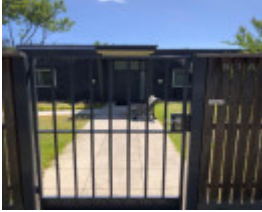
51A Union Street, Armadale
